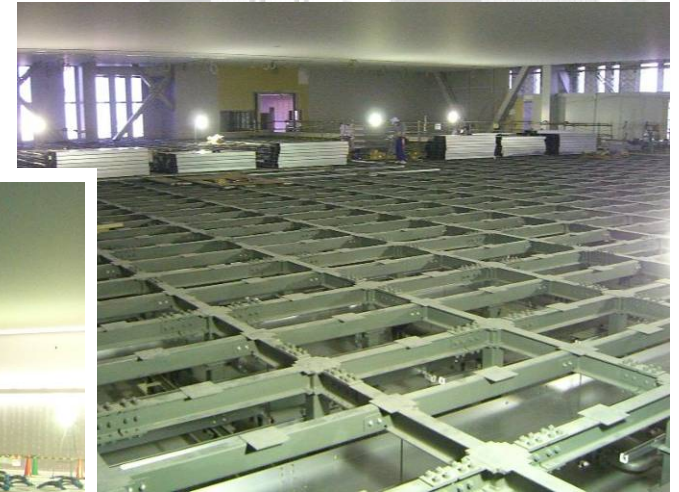
Making a double floor
